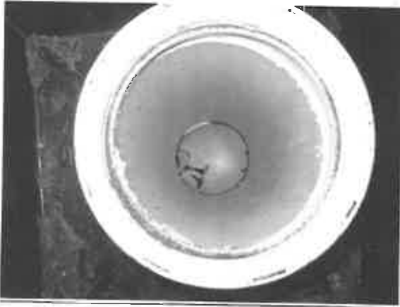
Figure 1 - View Inside Cleanout
