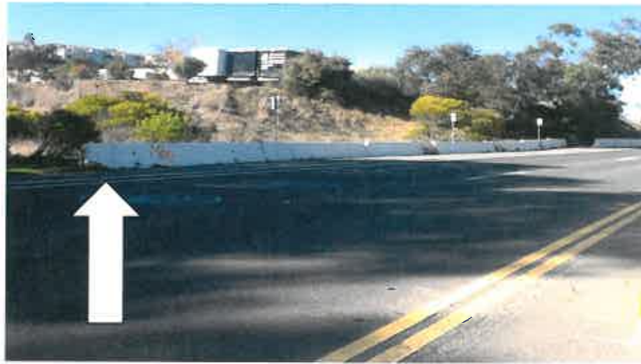
Access to former illegal dumping area restricted by k-rail
