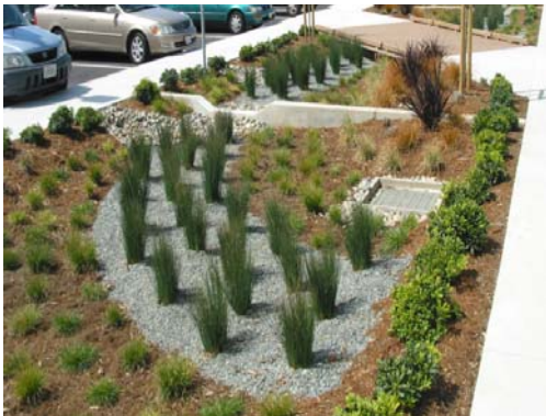
Bioretention Area, Brisbane
