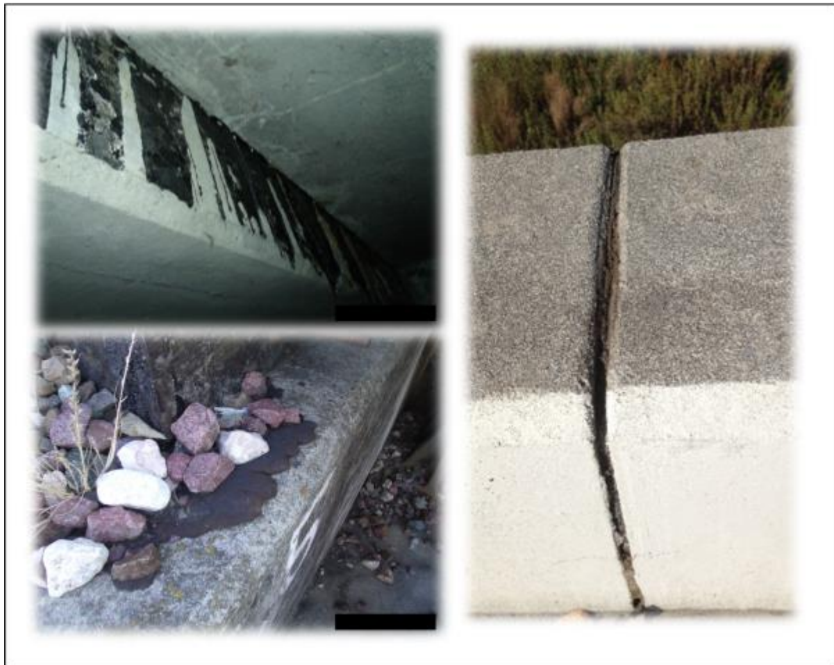
Figure 3.3 Examples of structures that were sampled and caulk or sealant materials that were included in the composites that had Low PCBs ( \geq 0.2 ppm and < 1 ppm). Not all structures or samples included in the Low PCBs category are pictured here.
