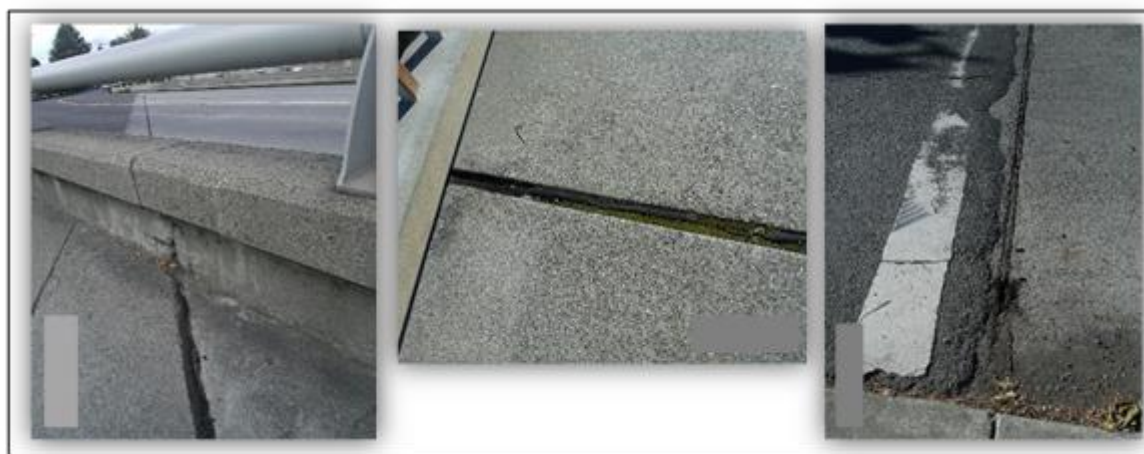
Figure 3.6 Examples of structures that were sampled and caulk materials that were included in Composite B, which had Very High PCBs ( \geq 1,000 ppm).
