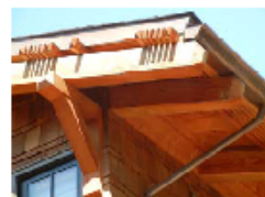
Building with copper flashing, gutter and drainpipe.
