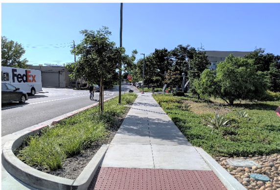
Figure 1-3: Stormwater planter at Independence Drive, Menlo Park
