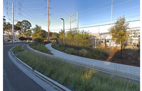
Figure 1-4 Stormwater planter at Chilco Street, Menlo Park
