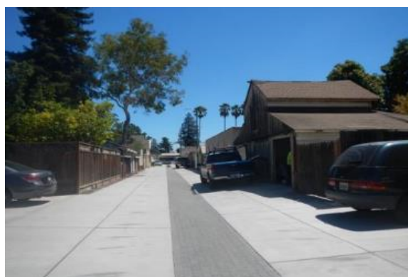
Figure 1-7 Infiltration trench, San Jose
