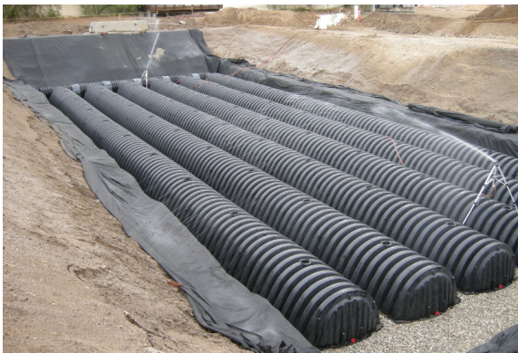
Figure 1-8 Subsurface Infiltration System example
