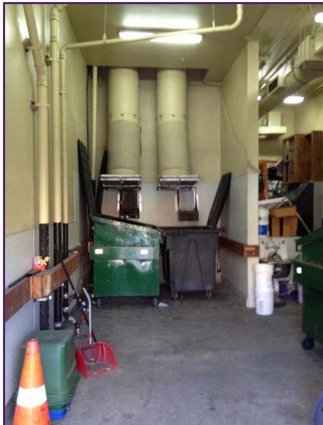
Figure 18. Trash room with dual chutes
