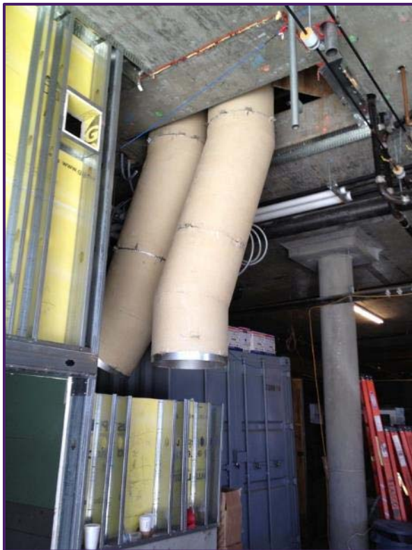
Figure 21. Problems during construction.
