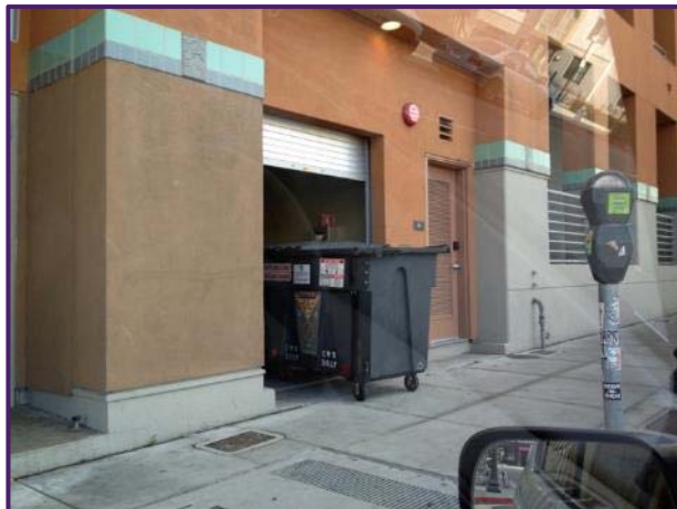
Figure 17. Access from chute room to street for hauler
