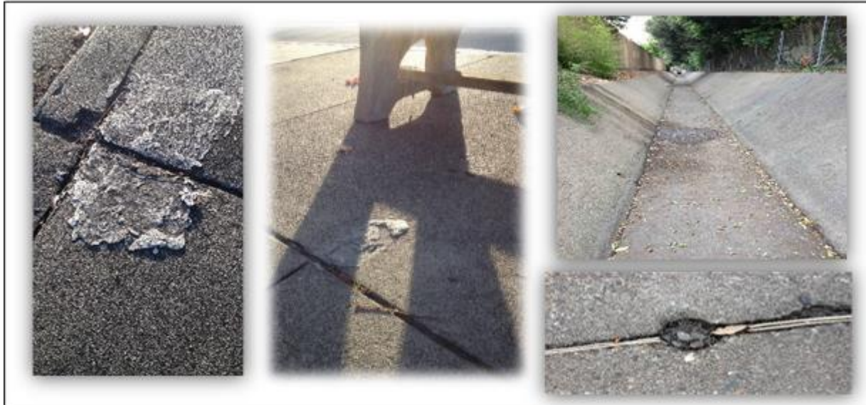
Figure 3.3 Examples of structures that were sampled and caulk or sealant materials that were included in composites that had Very Low PCBs (< 0.2 ppm). Not all structures or samples included in the Very Low PCBs category are pictured here.
