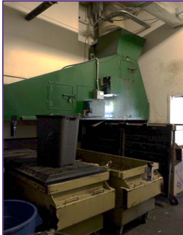
Figure 22. Final construction with Tri-Sorter.
