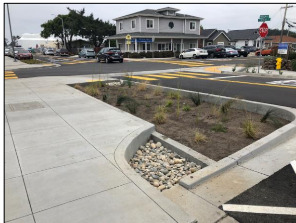
Figure 3-1. Completed Half Moon Bay Pilot
