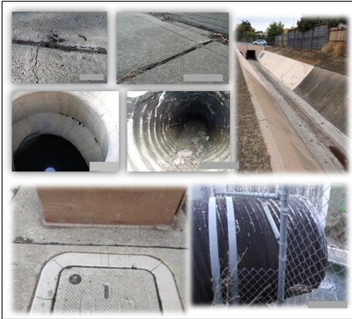
Figure 3.2 Examples of structures that were sampled and caulk or sealant materials that were included in the composites that had No PCBs Detected . Not all structures or samples included in the No PCBs Detected category are pictured here.
