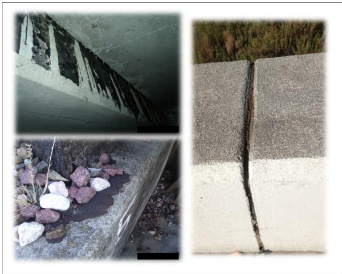
Figure 3.3 Examples of structures that were sampled and caulk or sealant materials that were included in the composites that had Low PCBs ( \geq 0.2 ppm and < 1 ppm). Not all structures or samples included in the Low PCBs category are pictured here.
