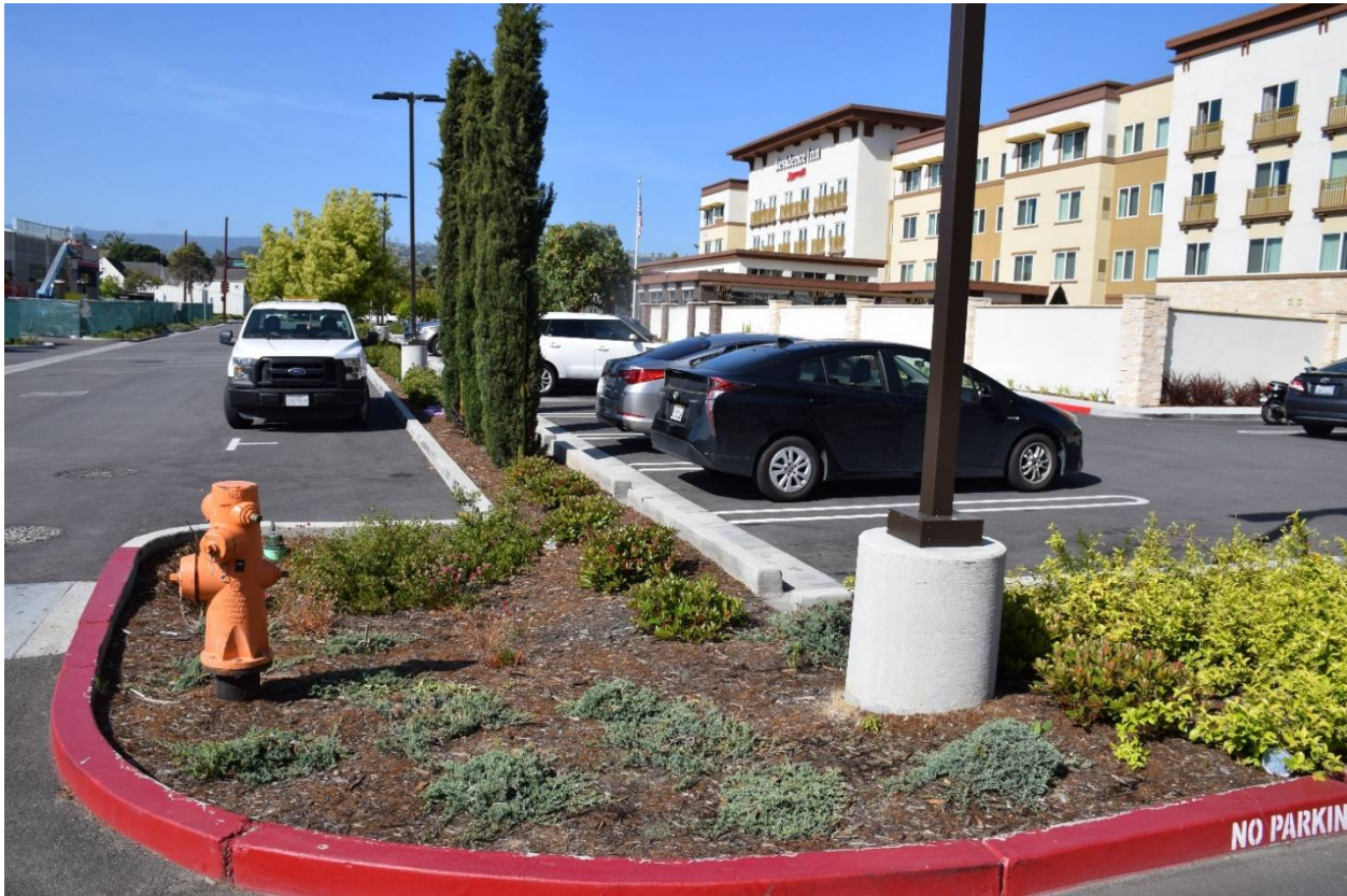
Bioretention area located at the Landmark Hotel.
