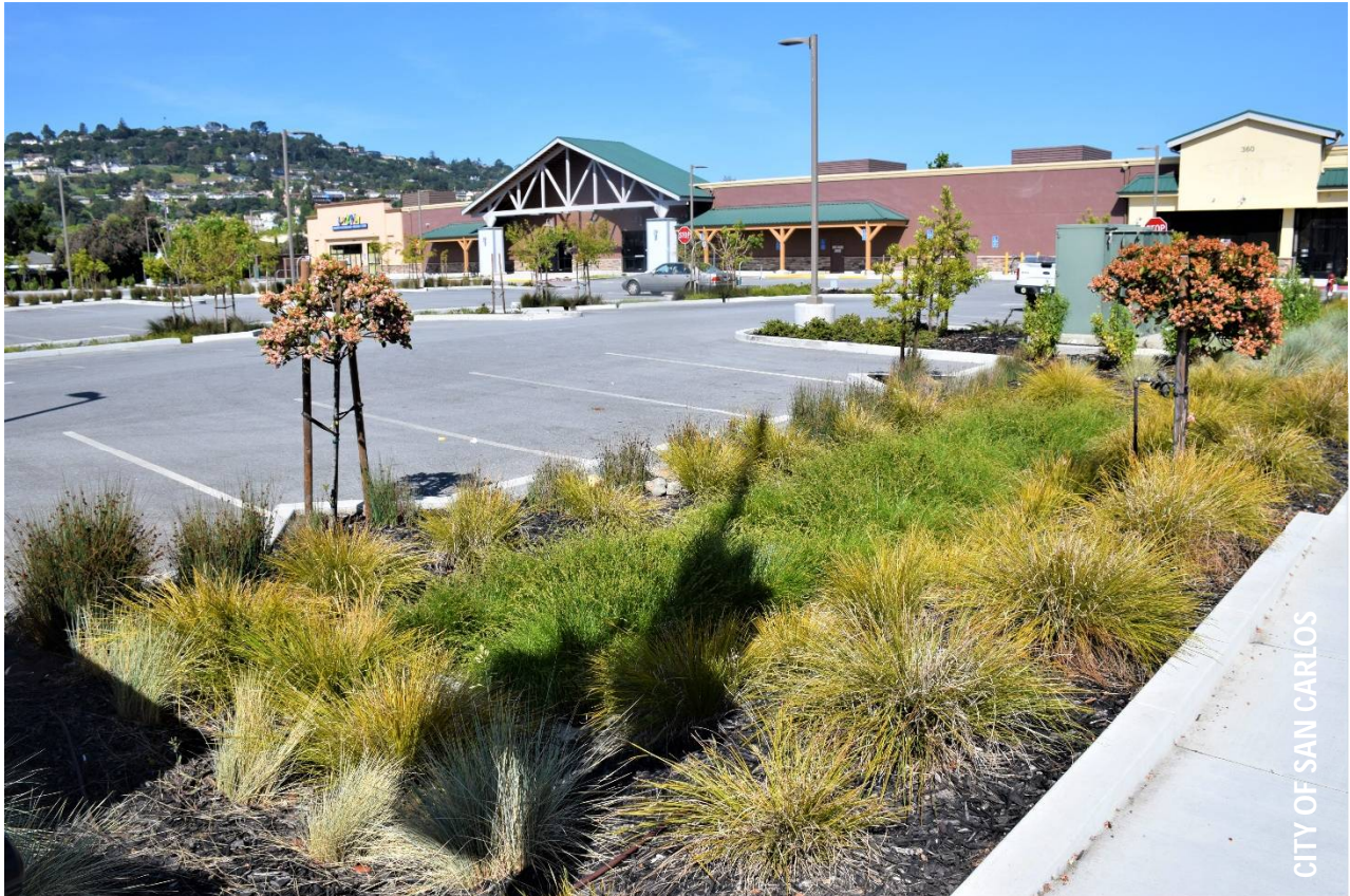
Bioretention area located at Orchard Supply Hardware Store.
