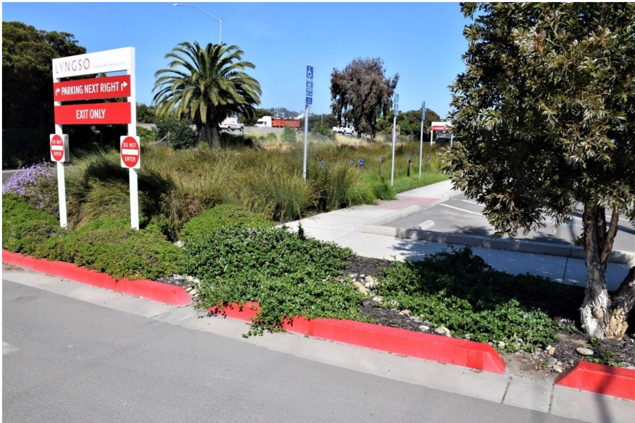
Bioretention area located at Lyngso on Shoreway Road.
