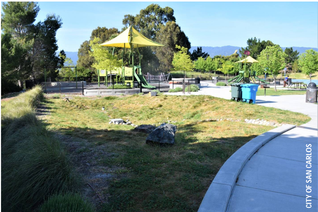
Bioretention area located at Crestview Park.
