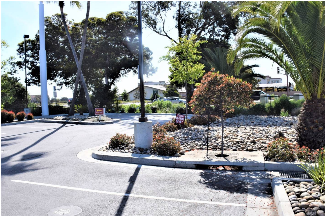
Stormwater tree well located at In-N-Out on Industrial Road.
