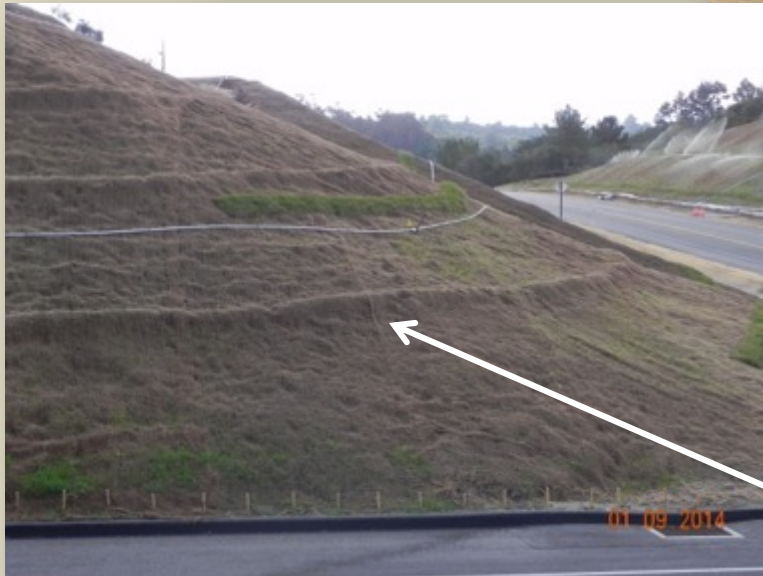
Netting installed over the compost berm
