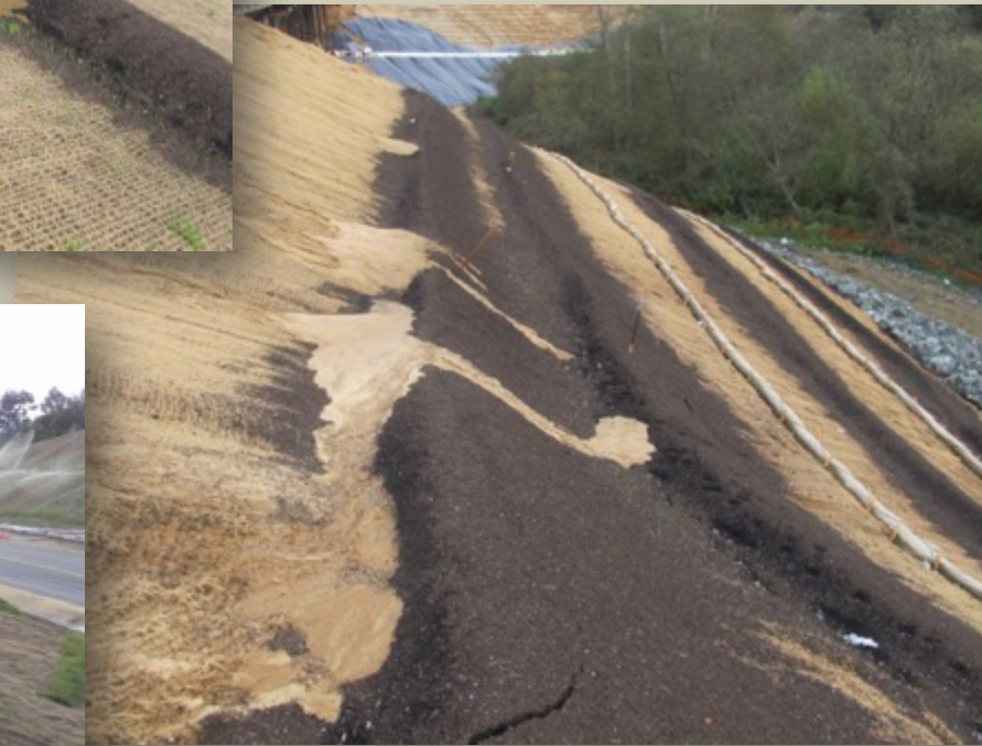
Netting installed over the compost berm
