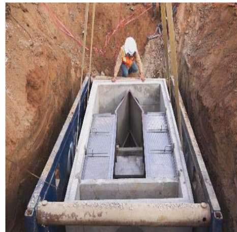
Figure 3-6. Two types of high-capacity trash full capture systems (HDS above, baffle box below).
