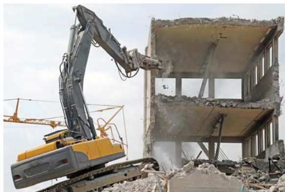
Figure 3-3. Demolition of a concrete slab building.
