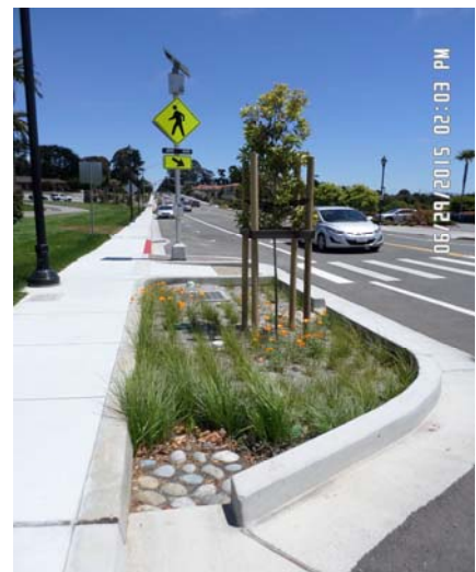
Figure 3-9. Hillside Boulevard green street project, Colma, CA.
