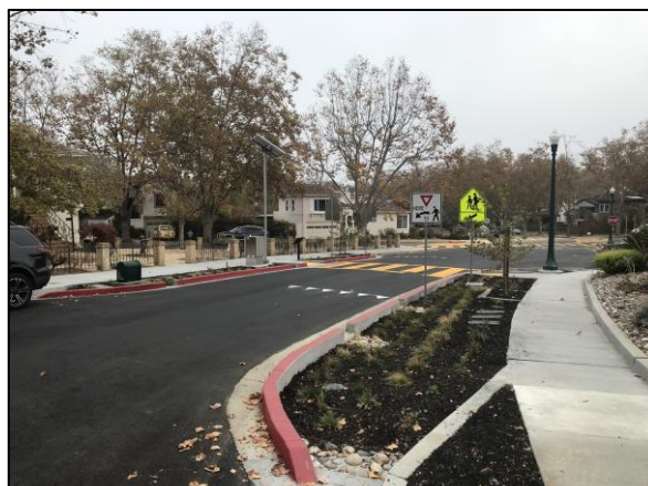
Figure 3-1. Completed Taylor Middle School Pilot Project, Millbrae
