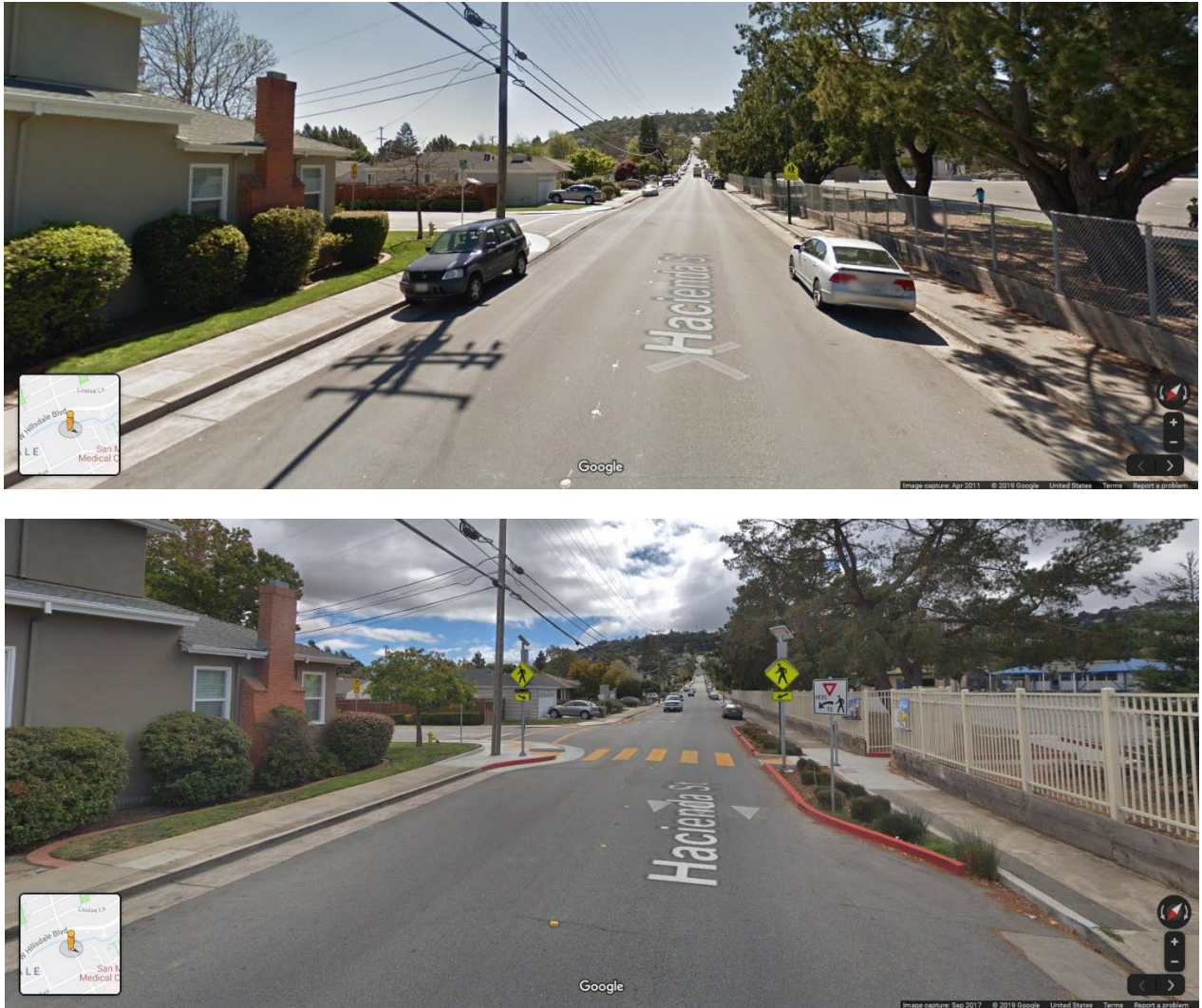
Figure 5. Example of Typology 1: Sustainable Street Curb Extension at a School Crossing in San Mateo
