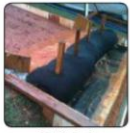
Fig. 2: 12" SiltSoxx™ (87% Removal Efficiency)
