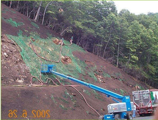
1:1 slopes with 'lock down' netting
