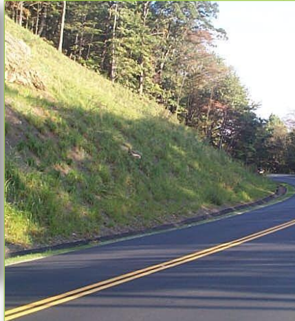
1:1 slopes with 'lock down' netting
