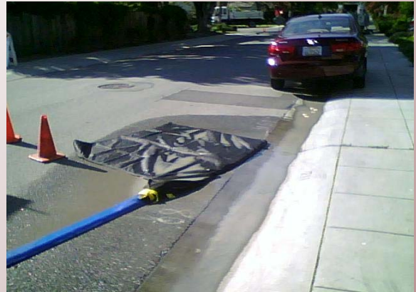
Filter bag w/dechlor tablets in gutter (Palo Alto WUDPPP)
