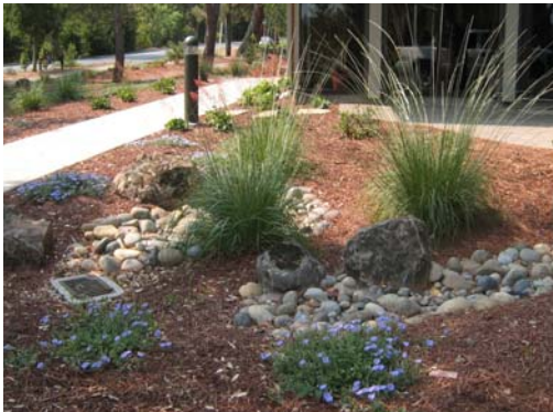
Landscaped area in a small project designed to receive runoff from the roof. (Photo credit: Stephanie Morris, landscape architect)
