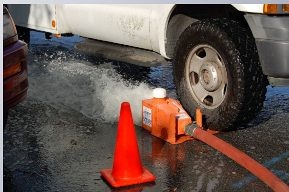
Diffuser (Palo Alto WUDPPP August 2011)
