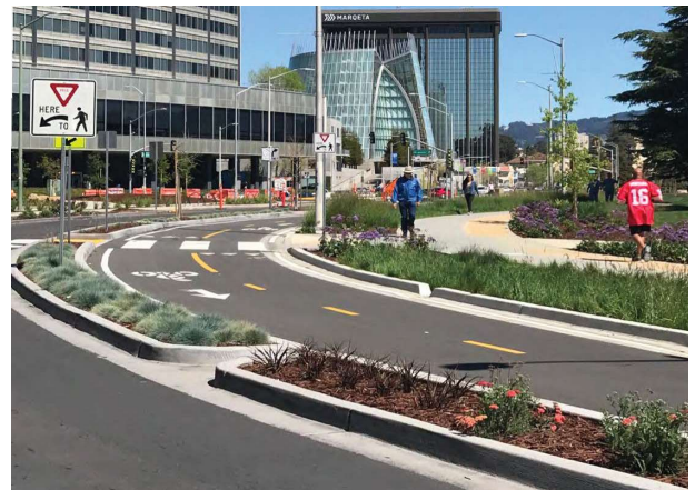
Photo 3: Stormwater planter, Harrison Street, Oakland Photo: CD+A
