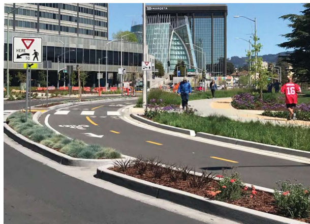
Photo 3: Stormwater planter, Harrison Street, Oakland Photo: CD+A
