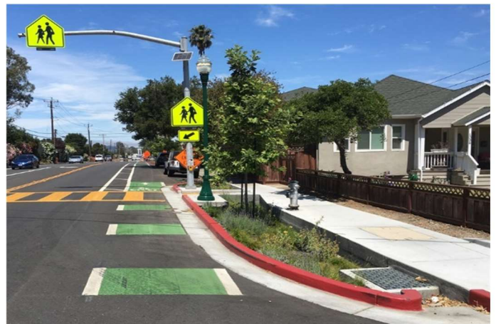
Photo 1. Bulb-out with raingarden in Burlingame, CA Photo: San Mateo Countywide Water Pollution Prevention Program
