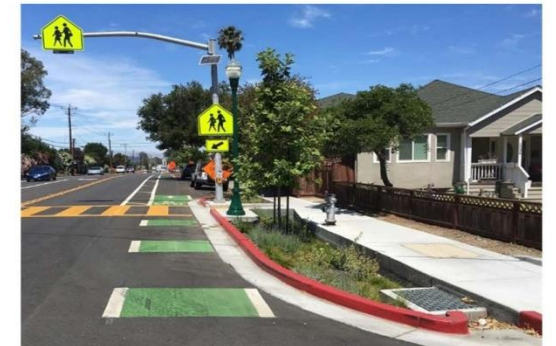
Photo 1. Bulb-out with raingarden in Burlingame, CA Photo: San Mateo Countywide Water Pollution Prevention Program
