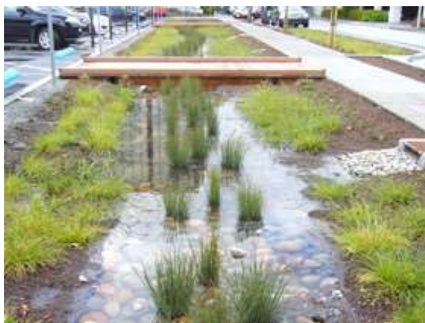
Photo 4: Rain garden and stormwater planters in curb extensions, Donnelly Avenue, Burlingame Photo: City of Burlingame
