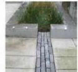
Open jointed paver water interception into a planted area
