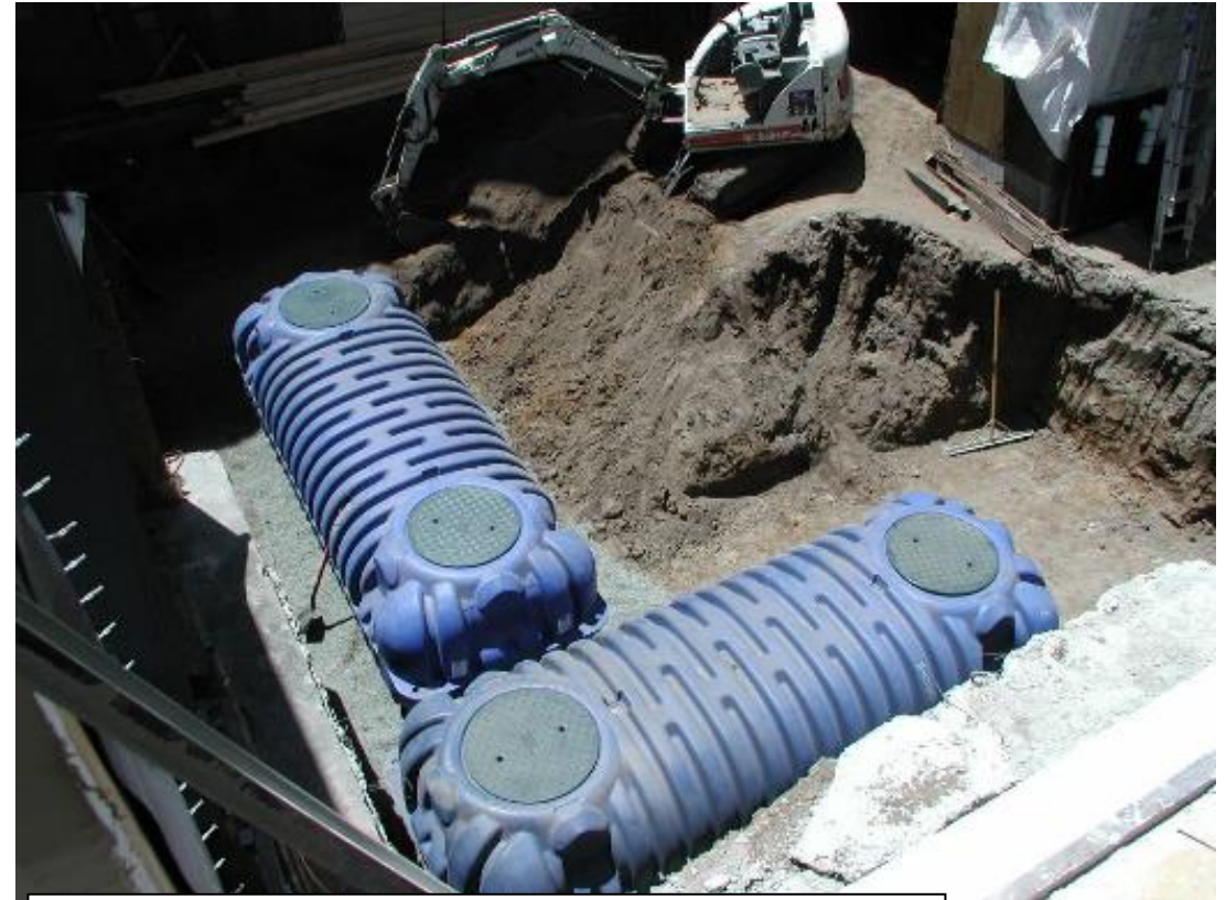
Cisterns installed underground
