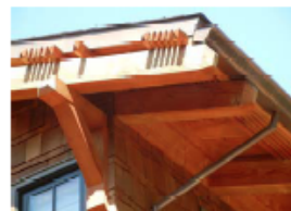
Building with copper flashing, gutter and drainpipe.
