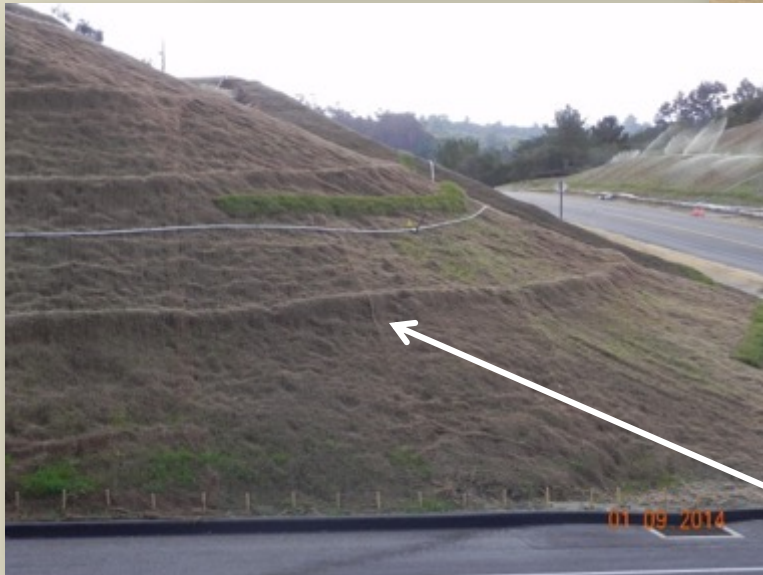
Netting installed over the compost berm
