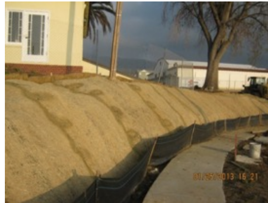
Examples of Bonded Fiber Matrix (BFM) and netting applications.
