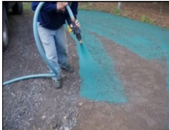
Examples of Bonded Fiber Matrix (BFM) and netting applications.
