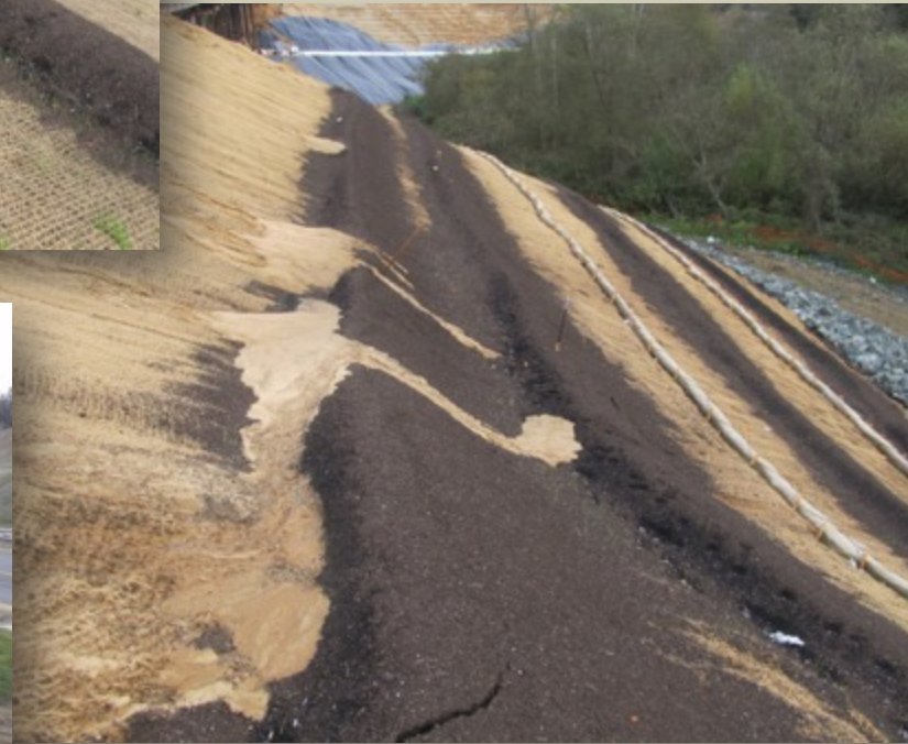
Netting installed over the compost berm
