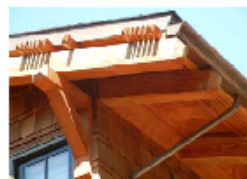
Building with copper flashing, gutter and drainpipe.
