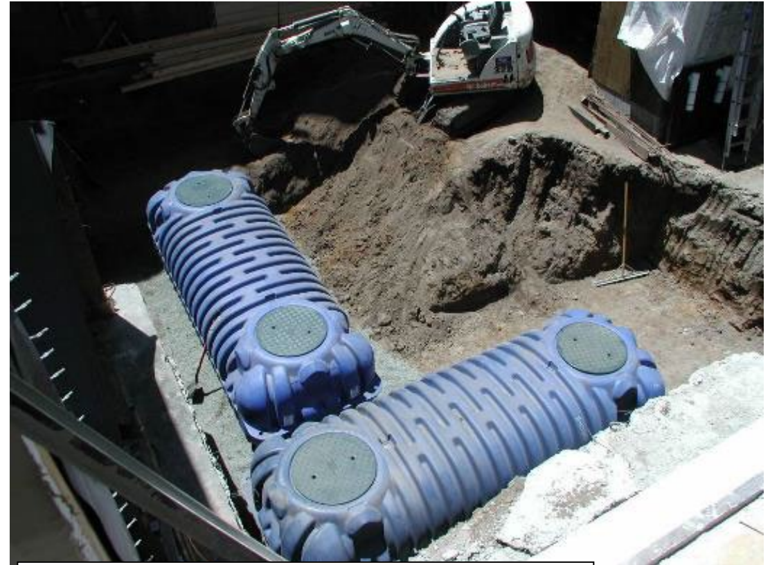
Cisterns installed underground
