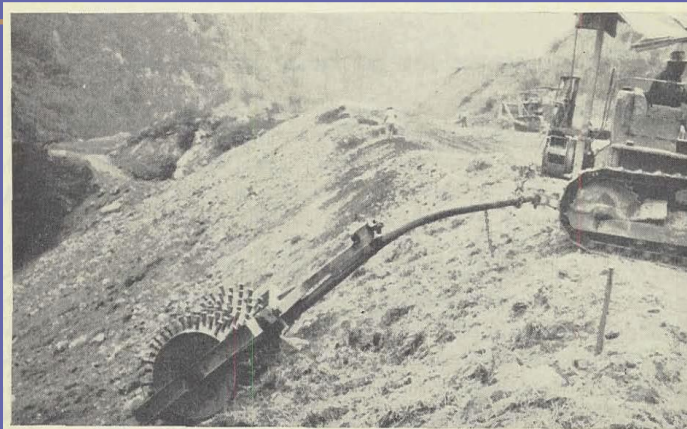
Rolling 10-foot strip of fill slope after application of straw. (City Creek Road, San Bernardino County)
