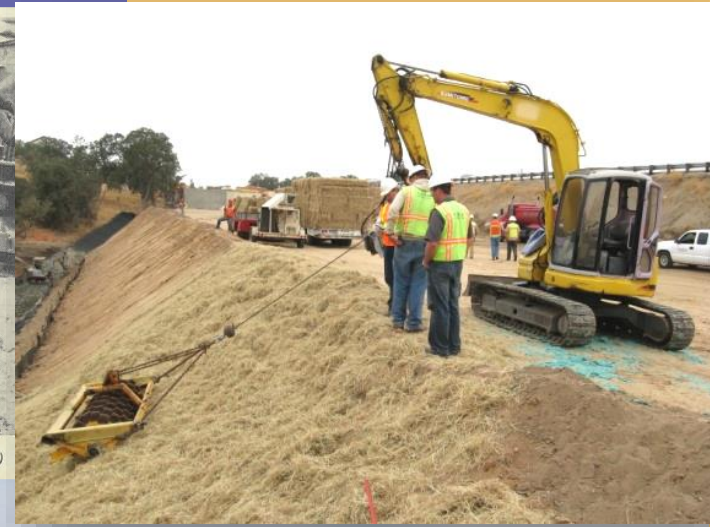
Rolling 10-foot strip of fill slope after application of straw. (City Creek Road, San Bernardino County)
