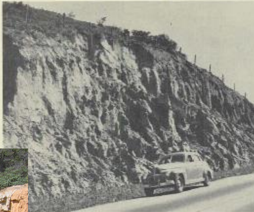
erode soil near Salinas. Note loss of soil above fence line. Sloped material way must be hauled away by truck
