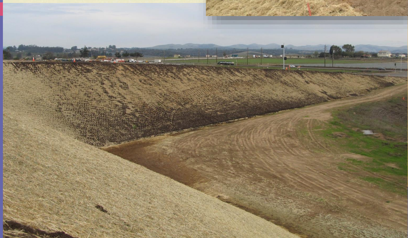
Rolling 10-foot strip of fill slope after application of straw. (City Creek Road, San Bernardino County)
