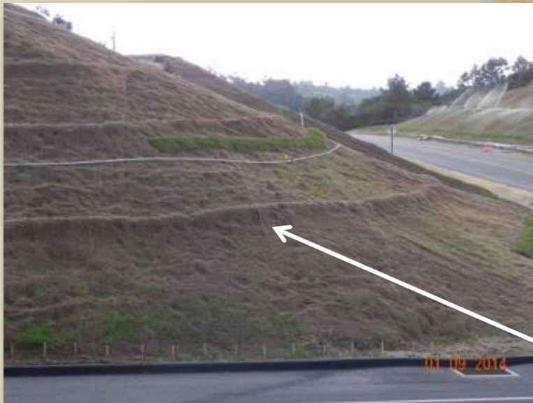
Netting installed over the compost berm
