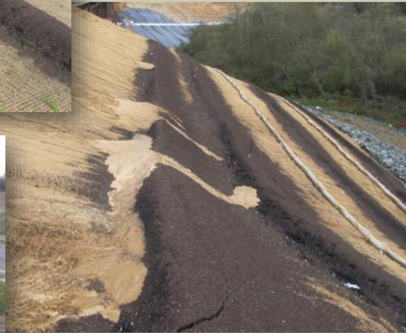
Netting installed over the compost berm
