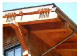
Building with copper flashing, gutter and drainpipe.
