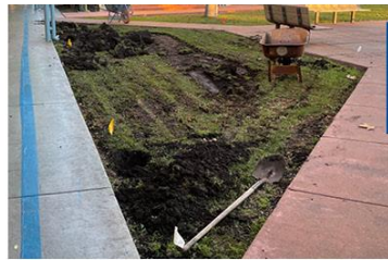
Excavation of the existing turf.
