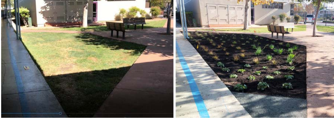
Figure 7-2. Before and after photo of the rain garden installed as part of the hands-on workshop.
