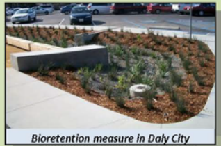
Bioretention measure in Daly City
