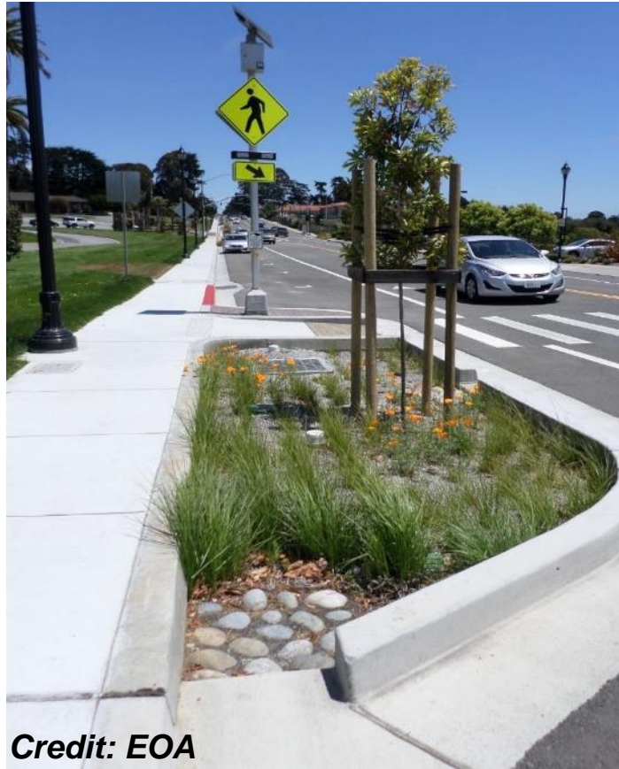
Stormwater Curb Extension
