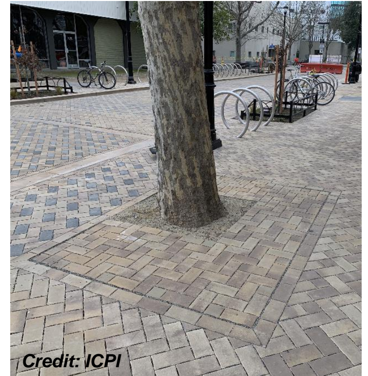
Tree Well Filter/ Pervious Pavement
