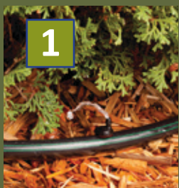
1 On-line drip emitter inserted into blank tubing
