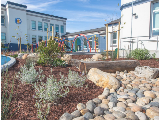
Stormwater bioswale as central feature in schoolyard
