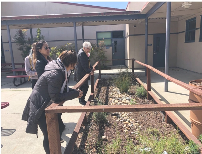
Demonstration stormwater garden in Quad
