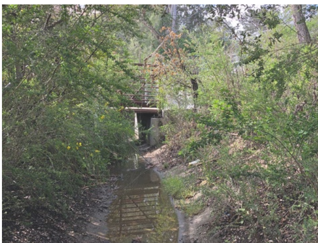
Creek at lunch area behind fence
