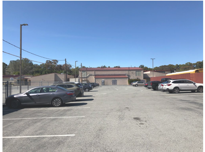
Parking on site looking towards gym
