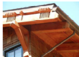
Building with copper flashing, gutter and drainpipe.
