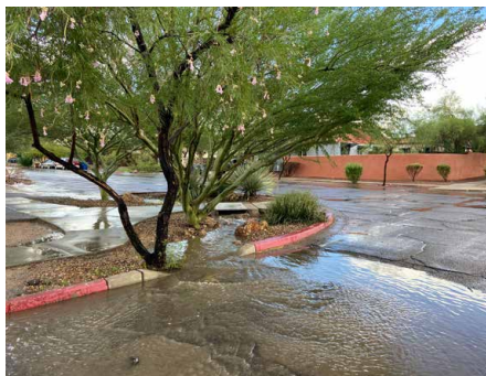
Photo Credit: City of Tucson, AZ
