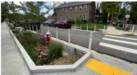
Street-scale facilities or “green streets”, such as curb extensions and bulb-outs designed to treat roadway runoff photo6
