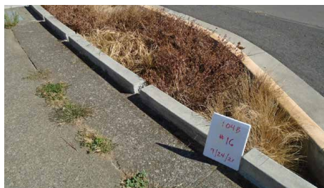
Impacts of June 2021 heat dome at a GSI facility without shade in the City of Portland. Photo Credit: City of Portland, OR, courtesy of Bureau of Environmental Services.
