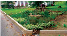
Parcel-based facilities, which are GSI measures sized to treat an entire parcel; and
