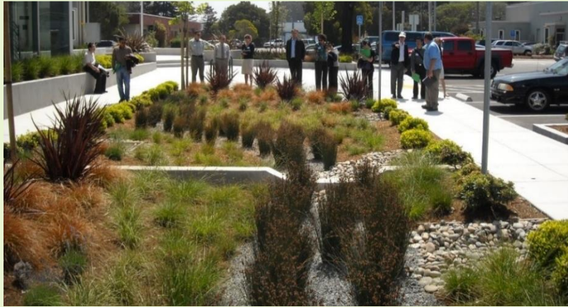
Figure 6-2: Bioretention area (Credit: City of Brisbane)
