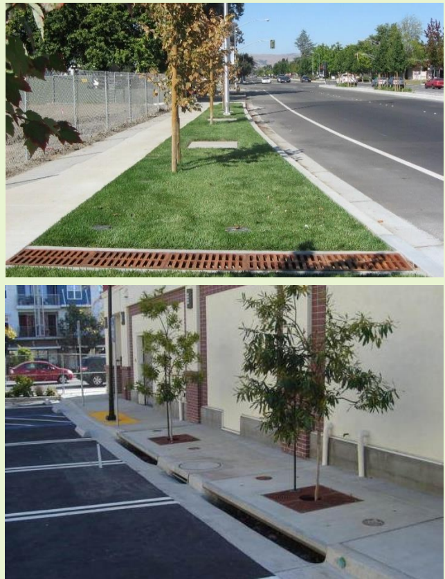
Figure 6-20: A tree well filter along a roadway (top – Credit: City of Fremont); and proprietary high flow rate tree well filters in a parking lot (bottom - Credit: City of Emeryville)
