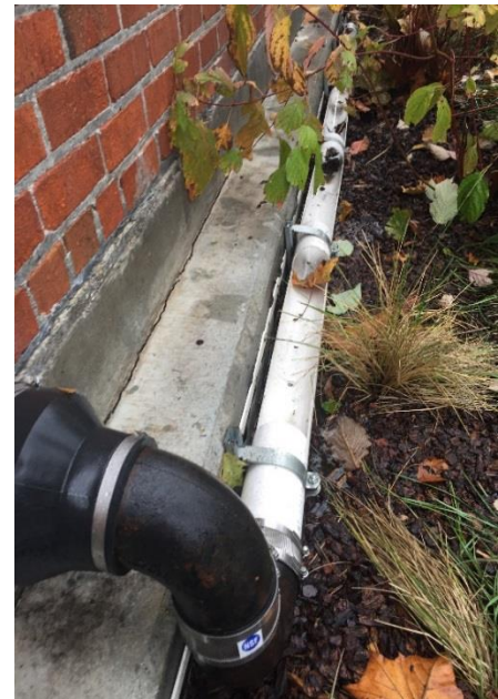
Figure 5-22: This flow-through planter has a flow spreader pipe to distribute water around the surface and away from the one inlet in the images. (Credit: EOA, Inc.)
