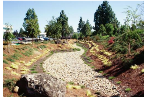
Figure 8-8: Extended Detention Basin, Palo Alto
