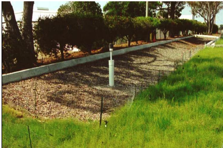
Figure 8-7: Infiltration Trench (Credit: CASQA)
