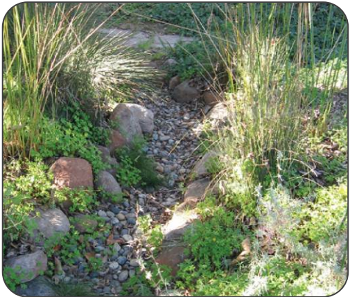
Dry creek infiltrates and conveys runoff.
