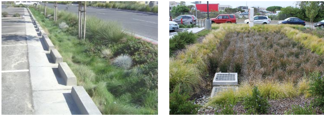
Figure B-2: Examples of Bioretention Areas
