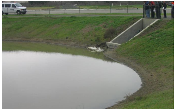
Figure 5-6: Detention pond used for hydromodification management.
