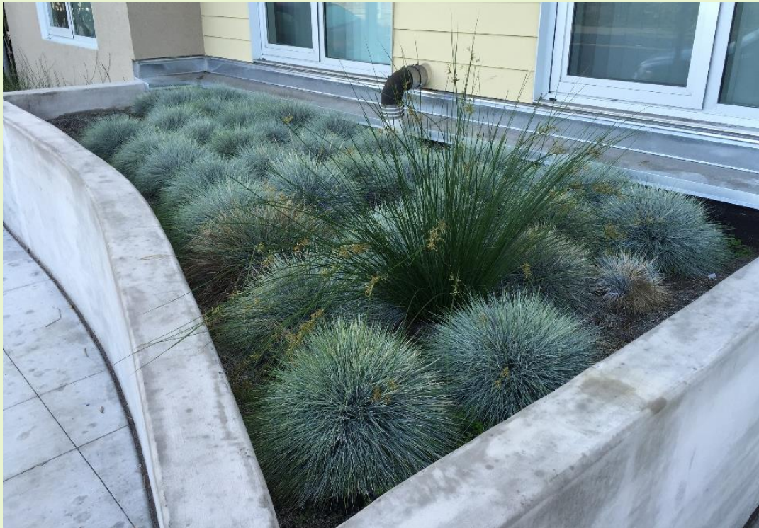
Figure 6-12: Flow-through planter (Credit: EOA, Inc.)
