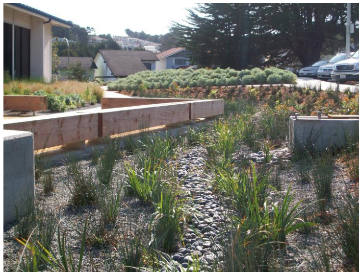
Figure 8-4: Bioretention Area in Daly City (Credit: SMCWPPP)
