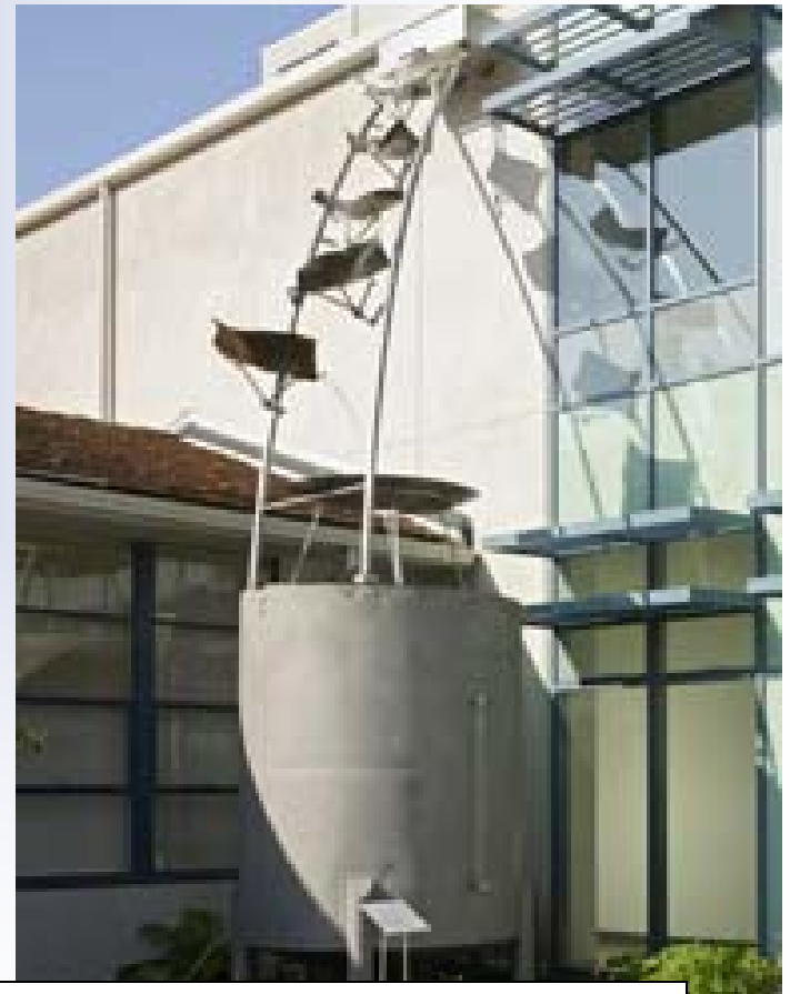
Harvesting for rainwater for indoor toilet flushing
