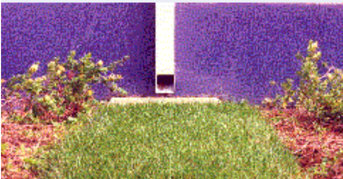
"Disconnected" downspout
