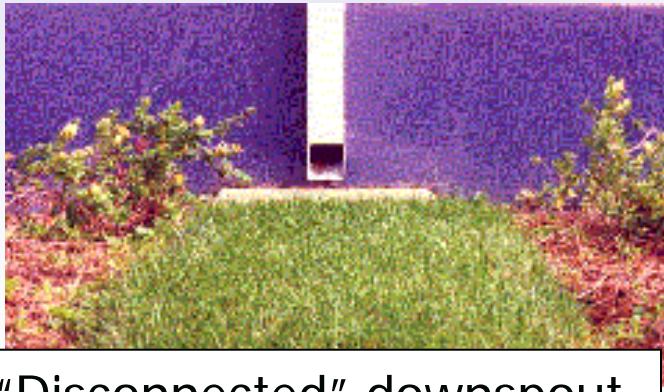
"Disconnected" downspout
