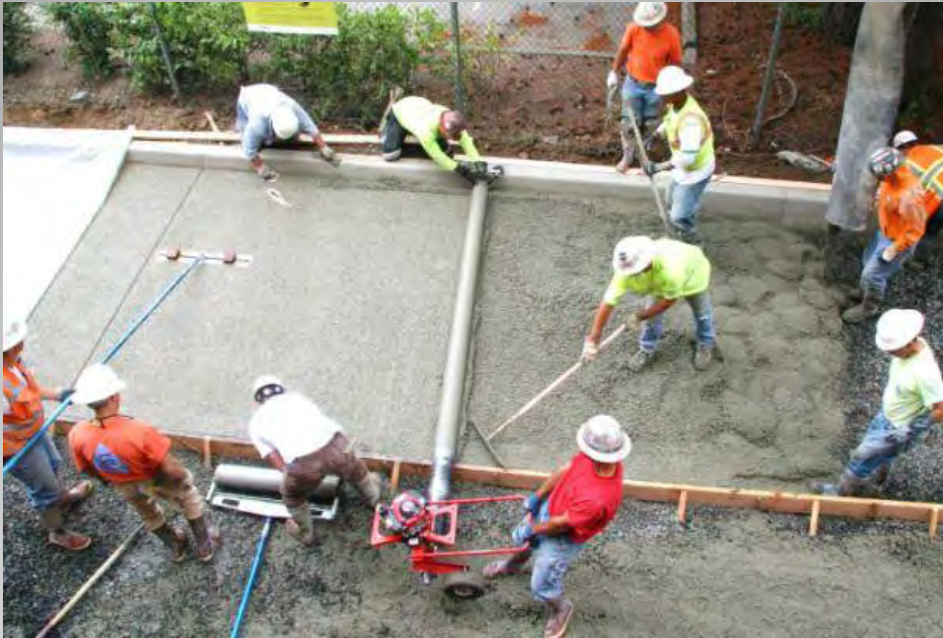
Pervious concrete being leveled & compacted w/ Bunyan Roller
