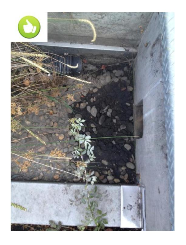
This Flow Splitter is designed to divert high flows from the system by using a weir inside the concrete box
