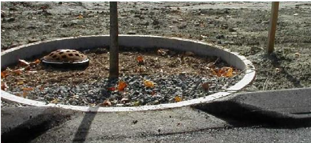
Figure 6-21: Tree well filter with curb-cut inlet. This tree well filter also features an overflow bypass (Source: University of New Hampshire Environmental Research Group, 2006)
