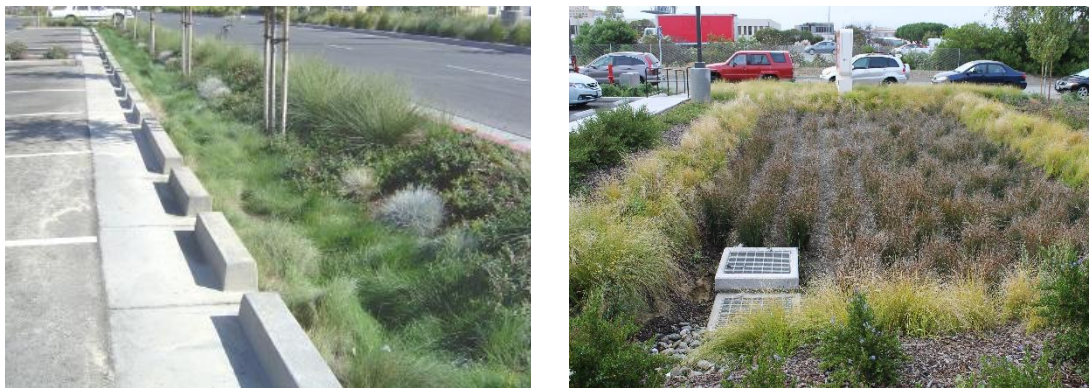
Figure B-2: Examples of Bioretention Areas
