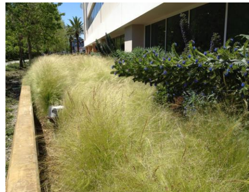
Figure 3-5: Flow-through planter in an urban setting (Credit: EOA, Inc.)
