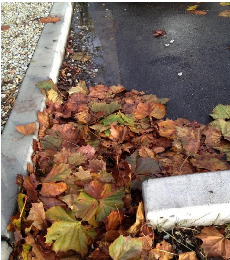
Figure 4-1. London plane tree leaves blocking an inlet (Credit: EOA, Inc.)
