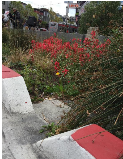
Figure 5-11: This standard curb cut in San Francisco has angled sides, a depressed throat and a 2-inch drop off to a splash apron. (Credit: EOA, Inc.)
