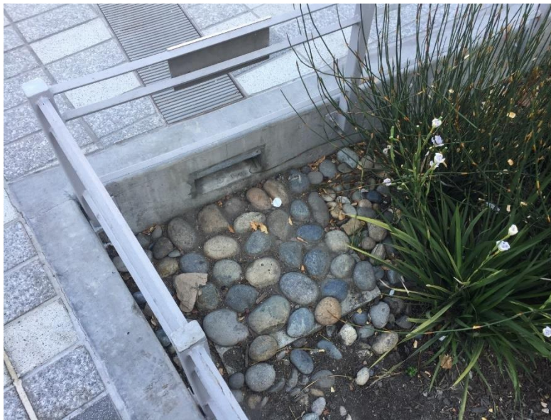
Figure 5-9: A concrete splash apron (with grouted cobble) is placed at the inlet to this stormwater treatment measure in Berkeley to help prevent erosion. Additional loose cobble is placed on the edges to prevent erosion. Other measures, such as using pea gravel or locating plants closer to the apron, could be used and would entail fewer maintenance issues than loose large cobble. (Credit: EOA, Inc.)
