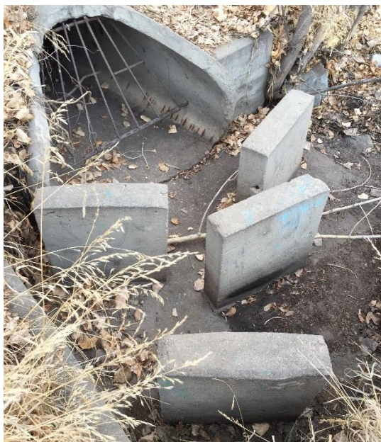
Figure 5-9: A concrete splash apron (with grouted cobble) is placed at the inlet to this stormwater treatment measure in Berkeley to help prevent erosion. Additional loose cobble is placed on the edges to prevent erosion. Other measures, such as using pea gravel or locating plants closer to the apron, could be used and would entail fewer maintenance issues than loose large cobble. (Credit: EOA, Inc.)
