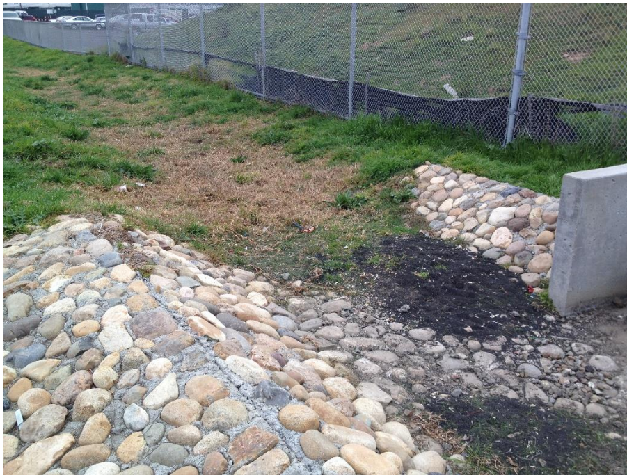
Figure 5-7: This bioretention area treats runoff from an artificial turf field in Berkeley and has an accumulation of crumb rubber particles (the black areas in the photo). (Credit: EOA, Inc.)
