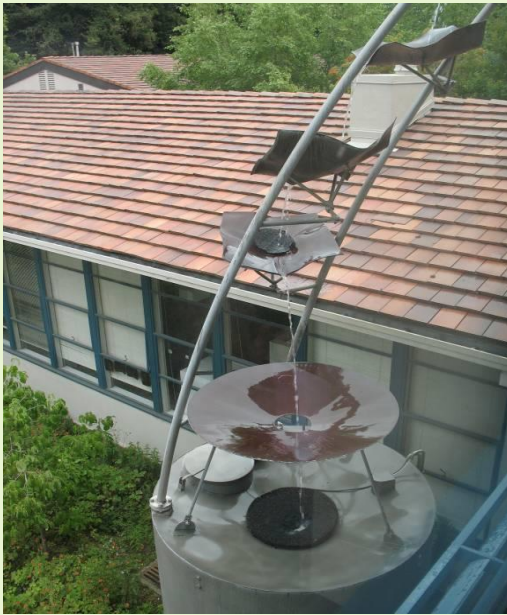
Figure 6-48: Rainwater is collected and used for flushing toilets at Mills College, Oakland. (Credit: EOA, Inc.)
