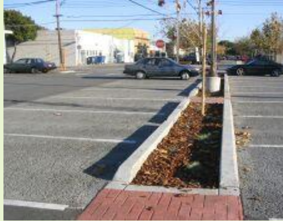
Figure 6-34: The City of Menlo Park used pervious concrete for parking stalls and standard paving in the drive aisles in this public parking lot. (Credit: City of Menlo Park)
