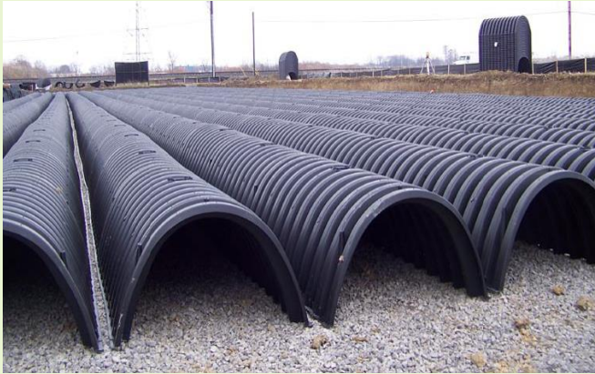
Figure 6-52: Photo of subsurface retention/infiltration system installation under a parking lot (Credit: CONTECH Engineered Solutions)
