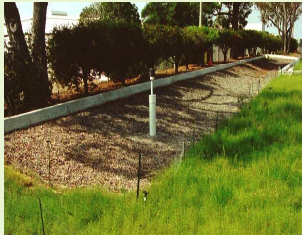
Figure 6-27. Infiltration Trench (Source: CASQA, 2003)
