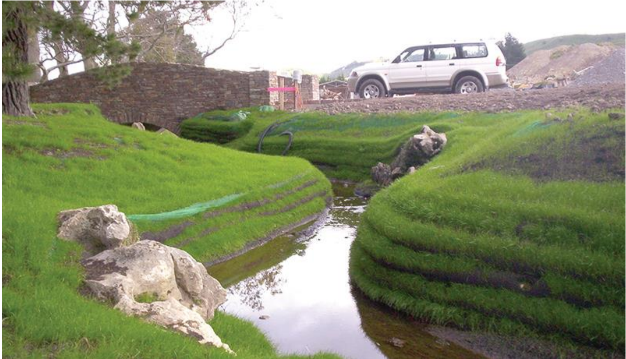
Figure 7-4: In-stream restorative measure using compost socks and vegetation (Credit: Filtrexx)
