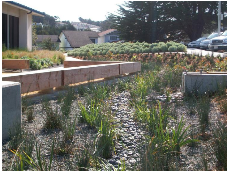
Figure 8-3: Bioretention Area in Daly City (Credit: SMCWPPP)
