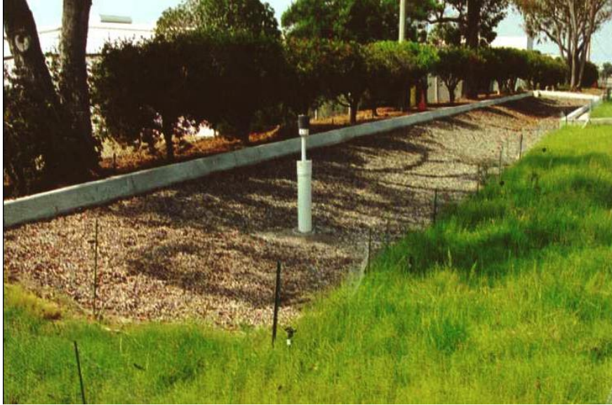
Figure 8-6: Infiltration Trench (Credit: CASQA)
