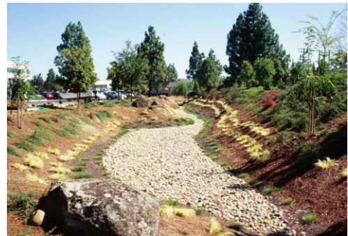
Figure 8-7: Extended Detention Basin, Palo Alto
