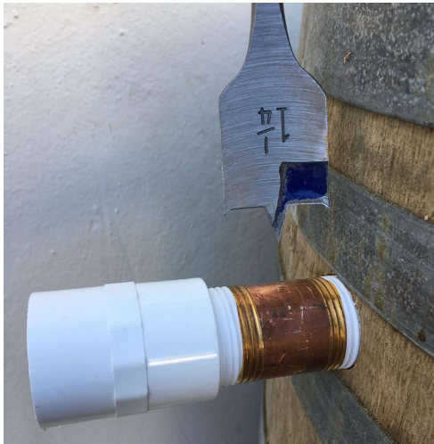
Figure 8. Overflow brass nipple sealed with teflon tape
