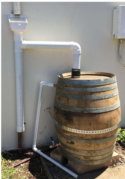
Figure 11. Finished product ready to catch rain!
